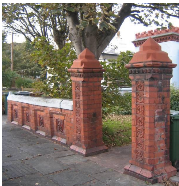
Boundary wall in brick and terracotta
