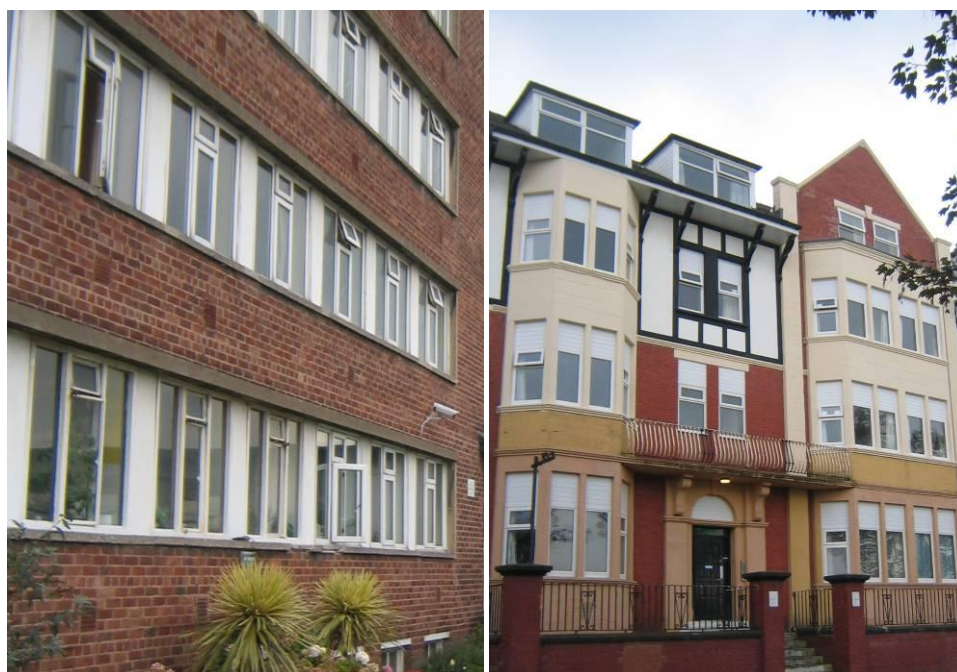
(left) Portland Court showing older steel glazing (bottom left) and newer uPVC units (elsewhere); (right) Marine Park Mansions, showing poorly proportioned dormers and reduced window heights.
